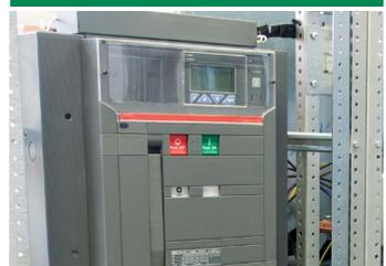
Sends trip signal to breaker trip coil (undervoltage or shunt trip) to interrupt power. Ability to trip upstream breaker if local breaker fails.
